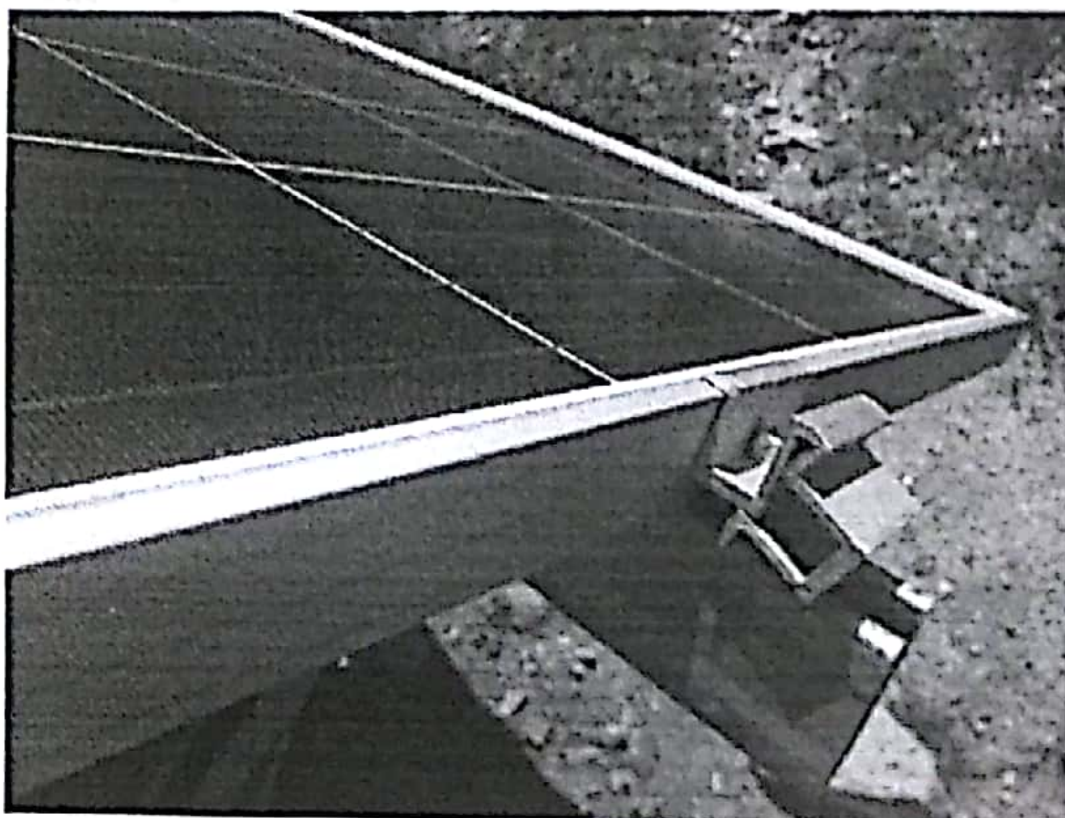
边压块用中压块代替、边压块安装歪斜不规范
