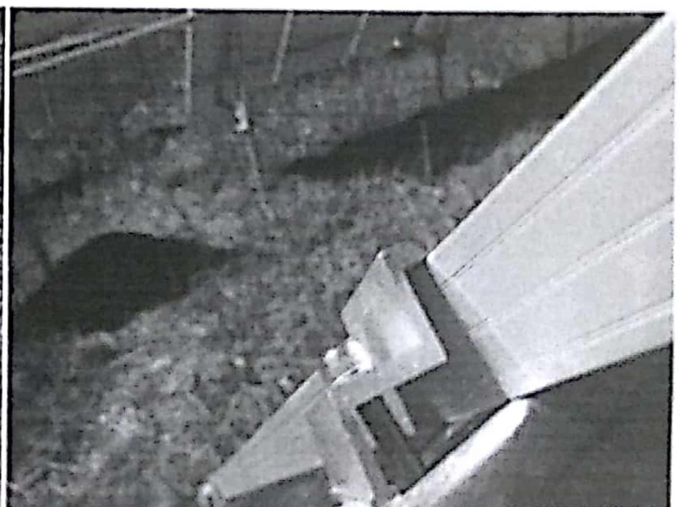
边压块用中压块代替、边压块安装歪斜不规范
