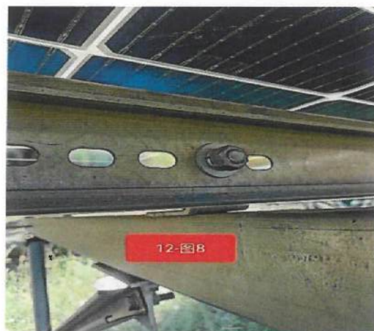
压块顶在光伏板上已整改
