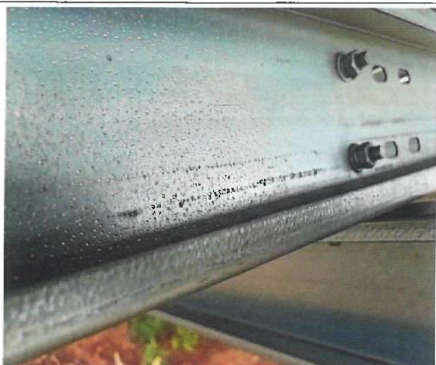
1 螺丝已加入垫片并紧固
