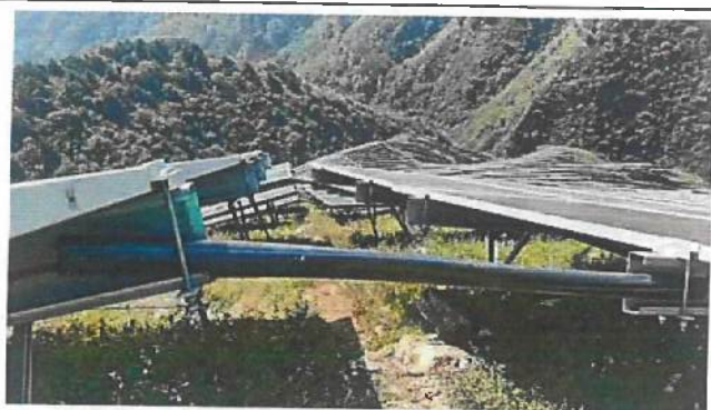
27 损坏套管已更换
