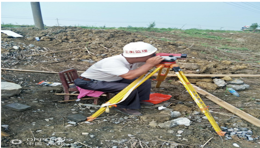
工地巡视六区检测桩标高、打桩 20170821
