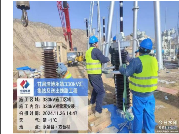
汇集站电气施工
