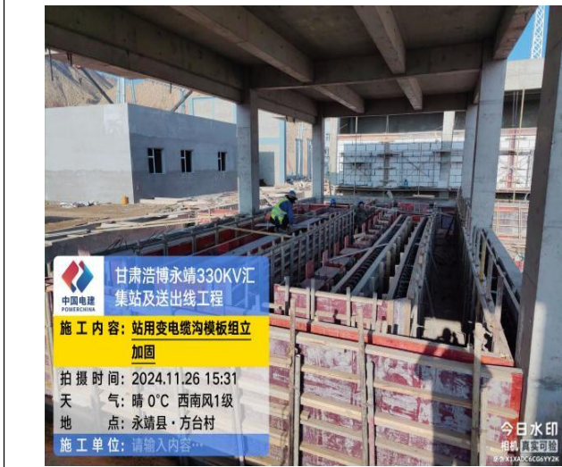
汇集站电缆沟施工
