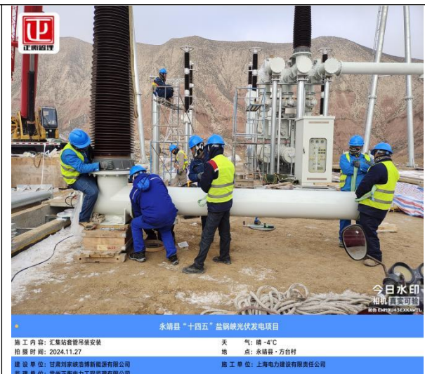
汇集站电气施工
