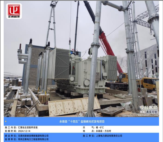
汇集站主变配件安装
