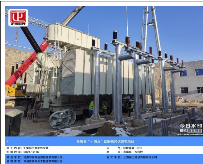
汇集站主变配件安装
