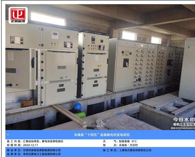
汇集站配电柜就位、放线
