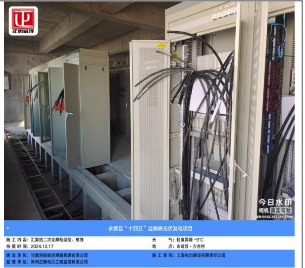
汇集站配电柜放线
