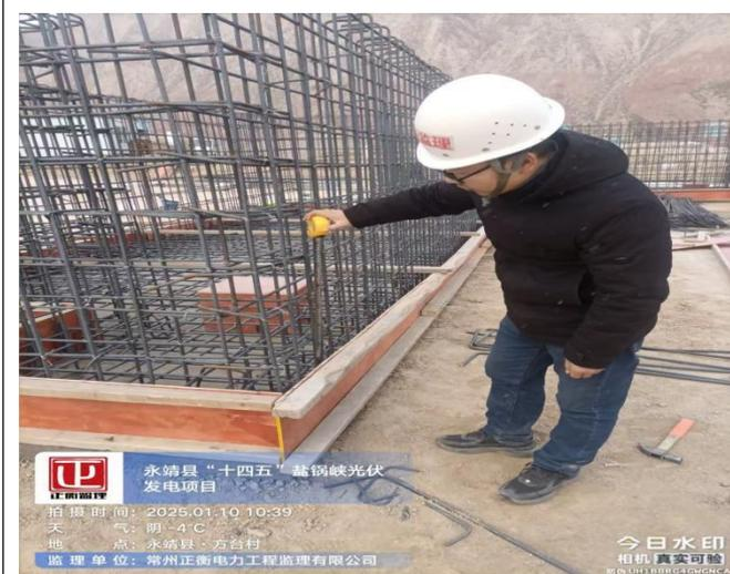
汇集站储能基础钢筋施工检查
