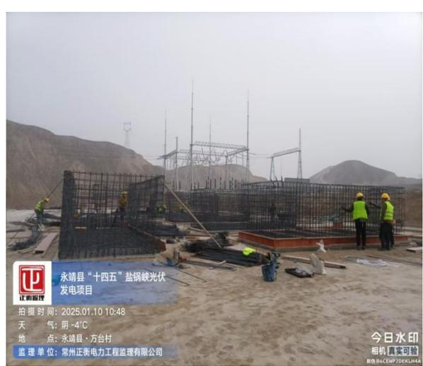
汇集站储能基础钢筋施工检查
