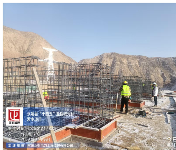
汇集站储能基础钢筋施工检查
