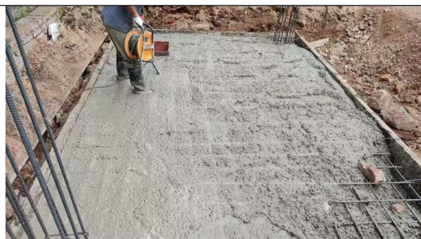
箱变基础底板浇筑振捣
