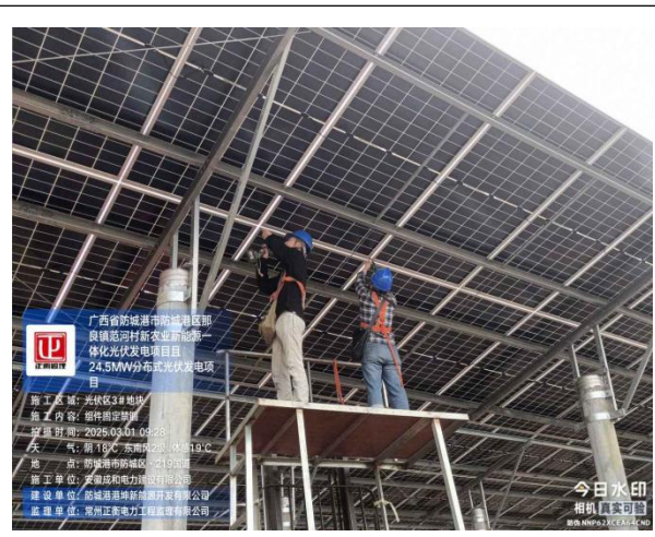
监理巡查三地块支架组件紧固
