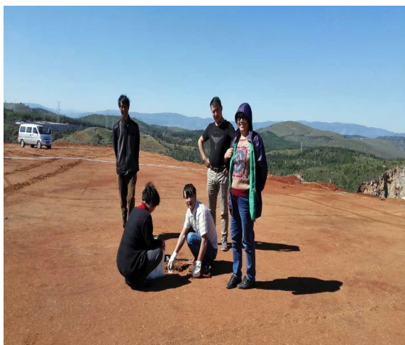
1#地块回填土环刀取样
