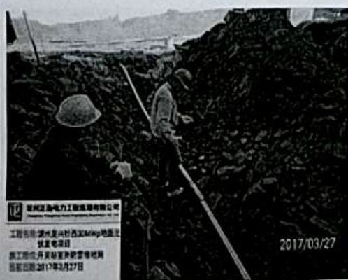
开关站室外接地网焊接
