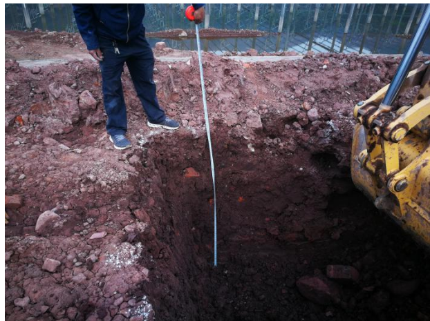
化粪池基坑开挖
