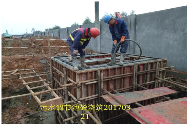
20170321 污水调节池砼浇筑
