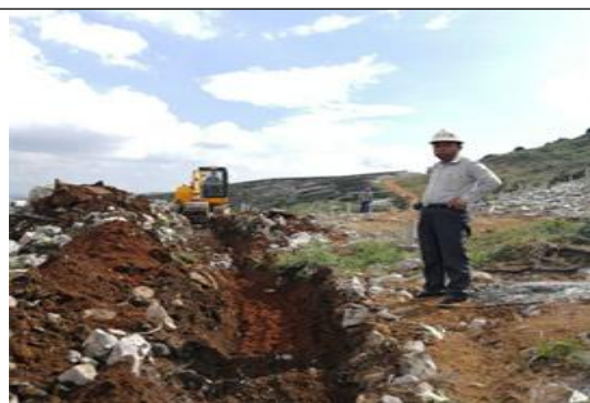
光伏东区21号方阵环形接地网沟土方开挖
