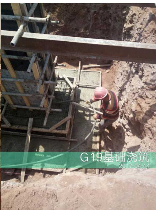
G19基础浇筑施工... 2017-04-14
