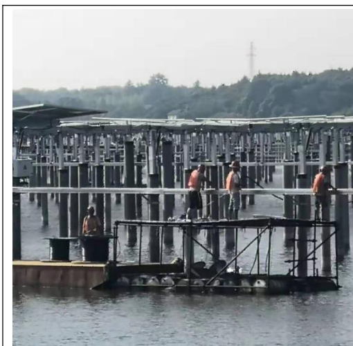
光伏区驱动机电源线敷设
