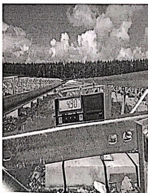
东区检测支架安装角度
