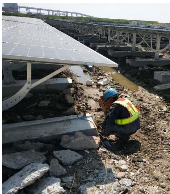
东区接地焊接敷设
