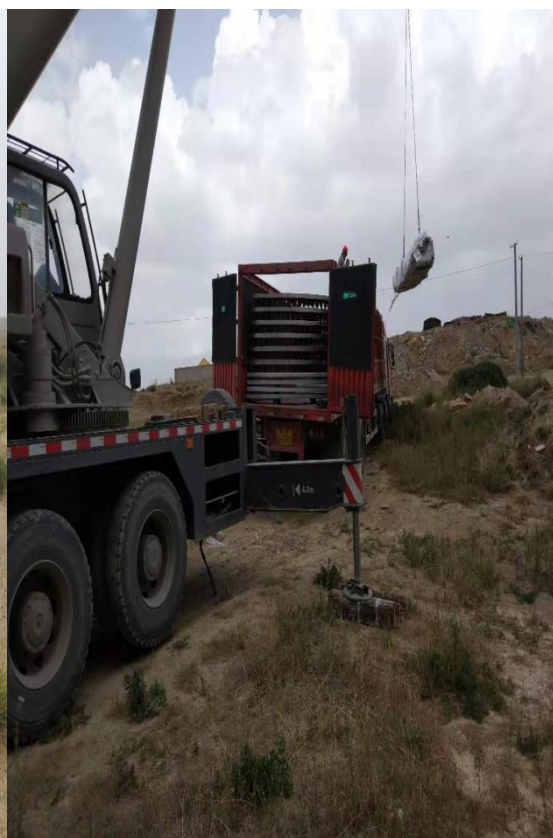
锚板进场卸货
