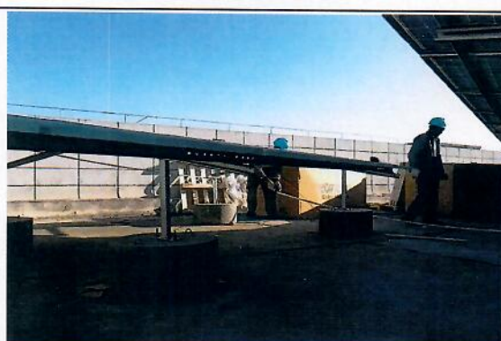
敷设低压电缆
