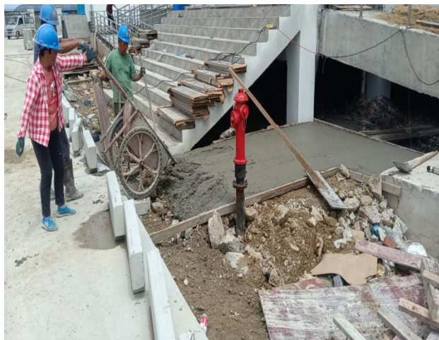
升压站人行道垫层浇筑
