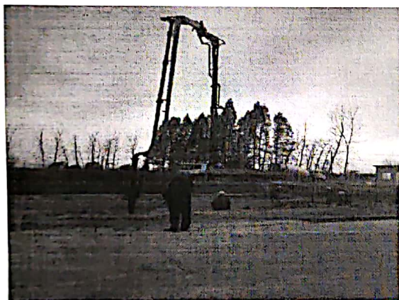
升压站基础垫层浇筑
