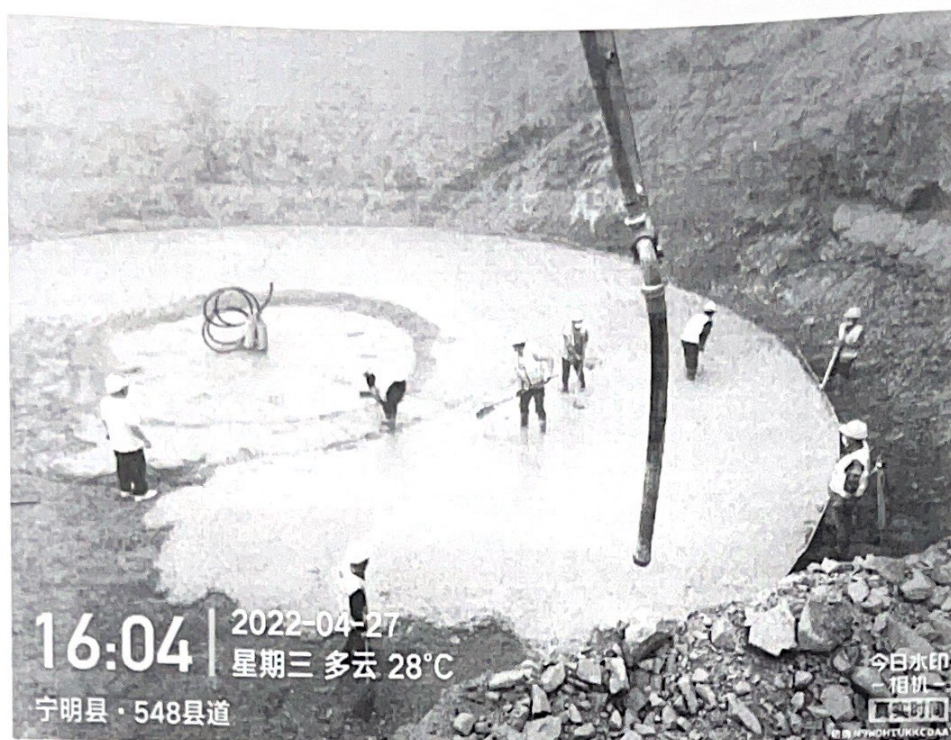
15#风机基础垫层浇筑
