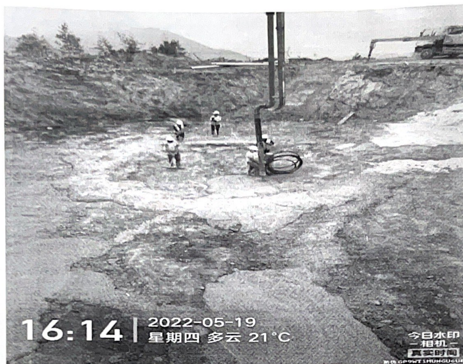
20#风机基础垫层浇筑
