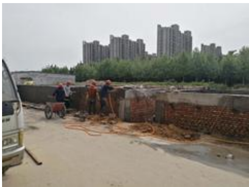
汇流开关站养护
