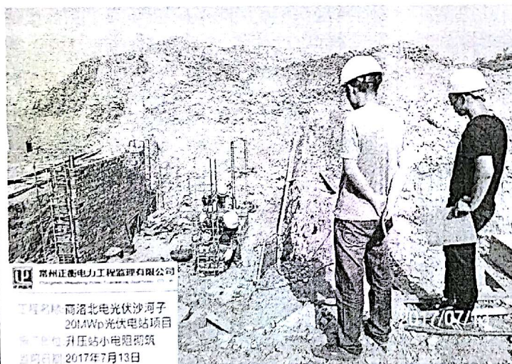
升压站小电阻砌筑
