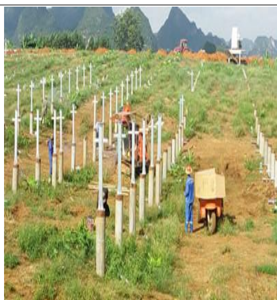
2 区预制桩立柱焊接
