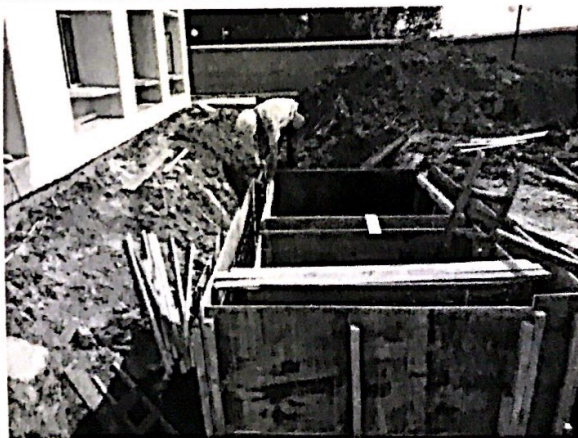
污水池基础支模
