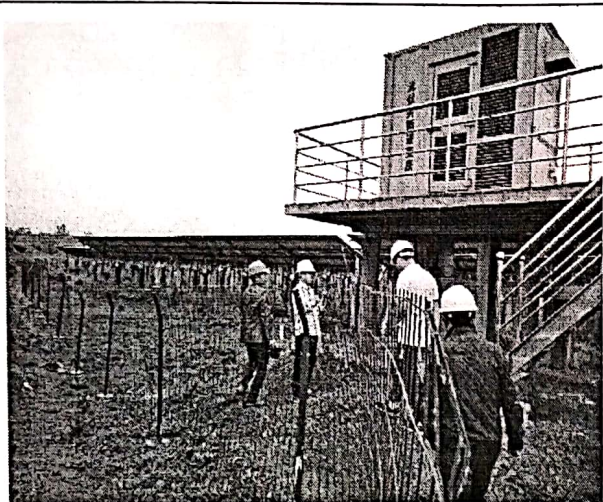
光伏 33 区检查验收
