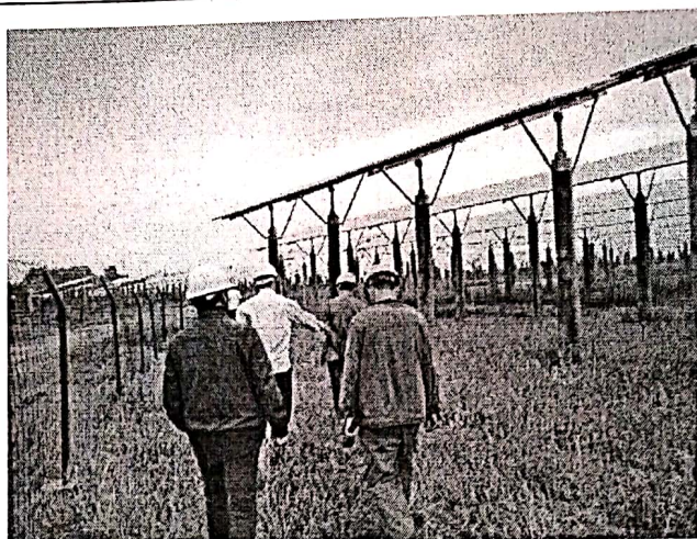
光伏 36 区检查验收
