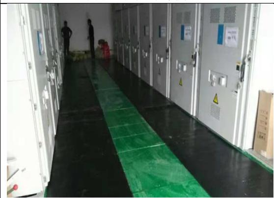
35KV配电室绝缘胶垫铺设
