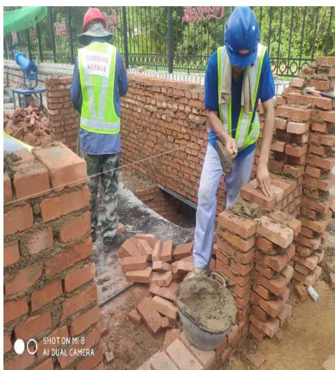
1#箱变基础砌筑
