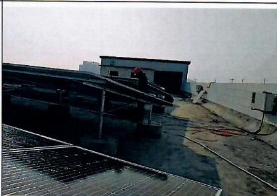
敷设低压电缆
