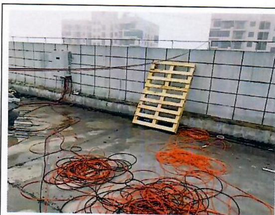
敷设低压电缆
