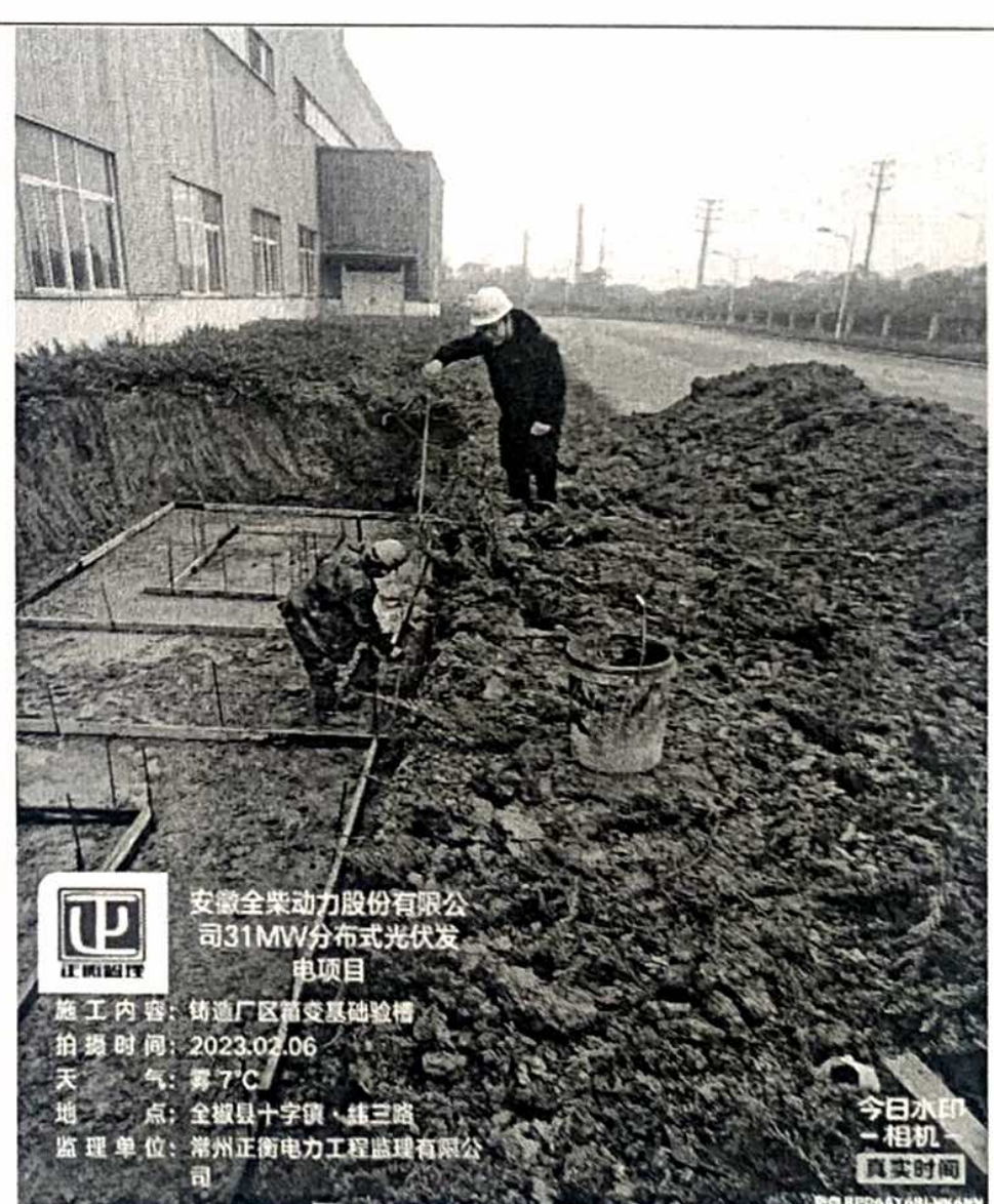
铸造厂区箱变基础验槽
