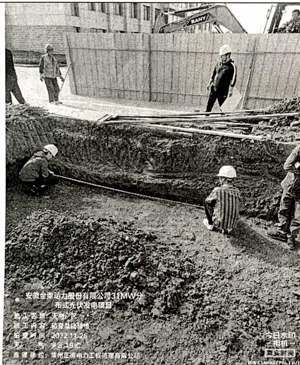
箱变基础验槽
