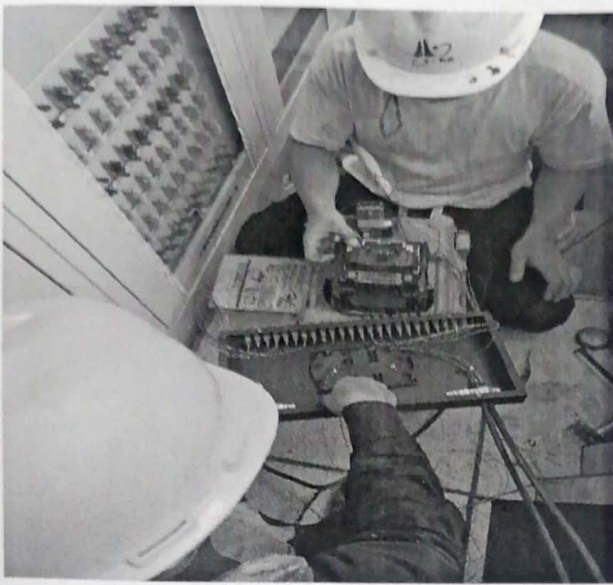
箱变环网光纤熔接
