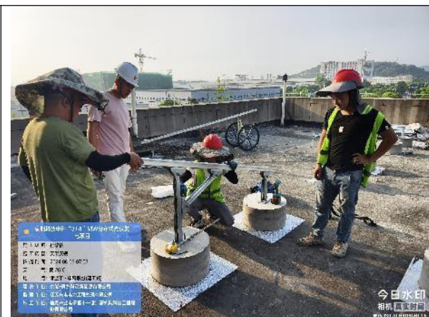
1#2#5#车棚基础开挖
