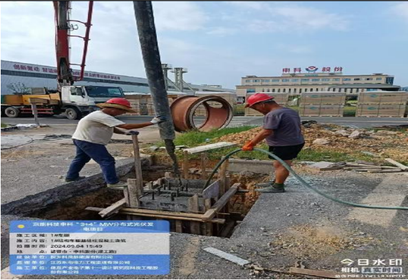
1#车棚短柱浇筑
