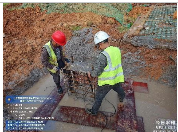
车棚基础地脚螺栓预埋
