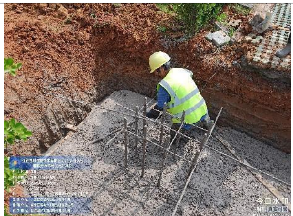
车棚基础地脚螺栓预埋
